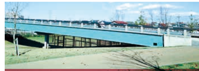
Over bridge A wide pedestrian bridge over the Seibu Line.
